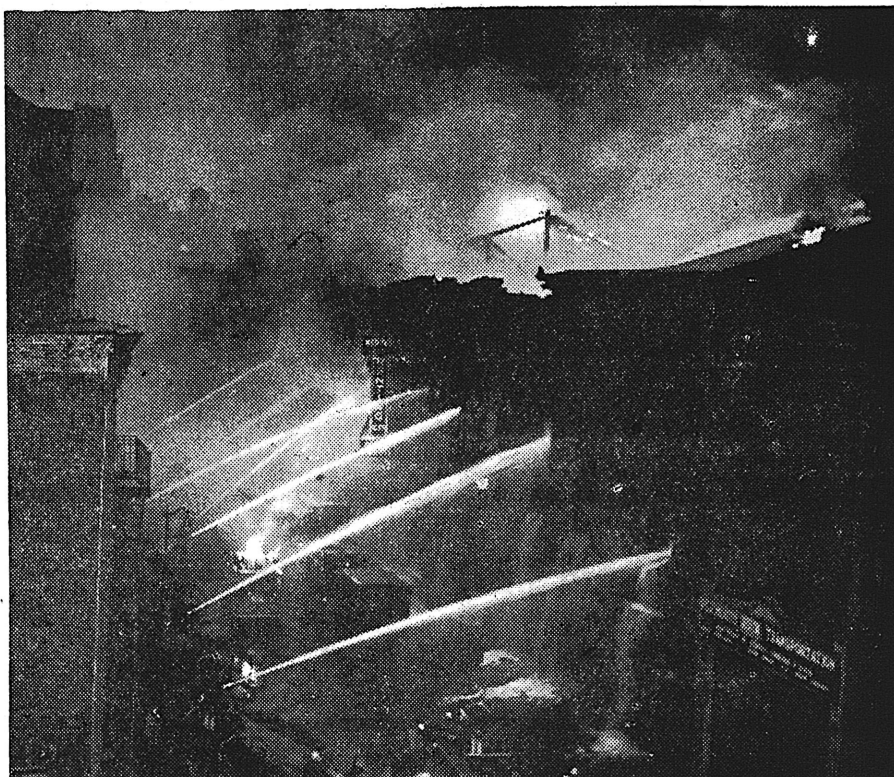
HUNDREDS OF VEHICLES GO UP IN SMOKE —Firemen played seven hoses into this garage in New York City in a futile effort to save an estimated 250 cars and trucks that were stored. The fire broke through the roof of the structure and gutted the building.
