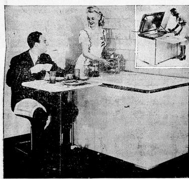
A new home freezer described as a "complete kitchen unit" has been announced by The Maytag Company of Newton, Iowa. With six net cubic feet of locker storage space and a capacity of 300 lbs. of meat or 240 lbs. of mixed packages, it maintains an operating temperature of zero Fahrenheit in all climates. When closed it provides a porcelain enamel utility table top with attached drop leaf for dinette purposes, large enough for two people. Inset shows counter-balanced lid opened
