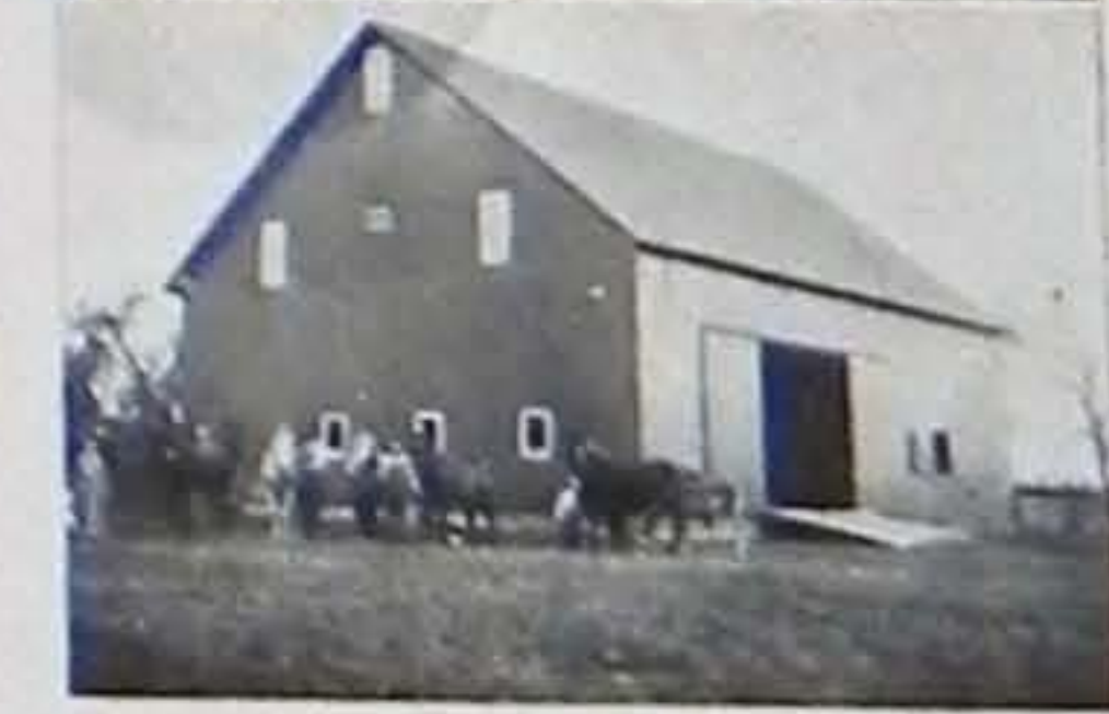
RESIDENCE AND BARN OF J. A. POUND, ARTHUR, ILL.
