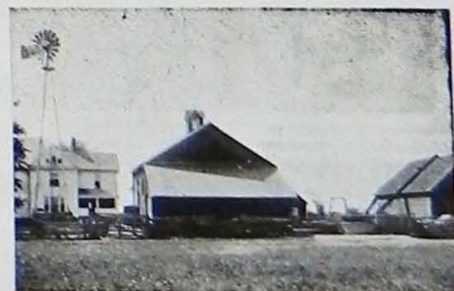
FARM BUILDINGS OF D. E. FREELAND, WINDSOR, ILL.
