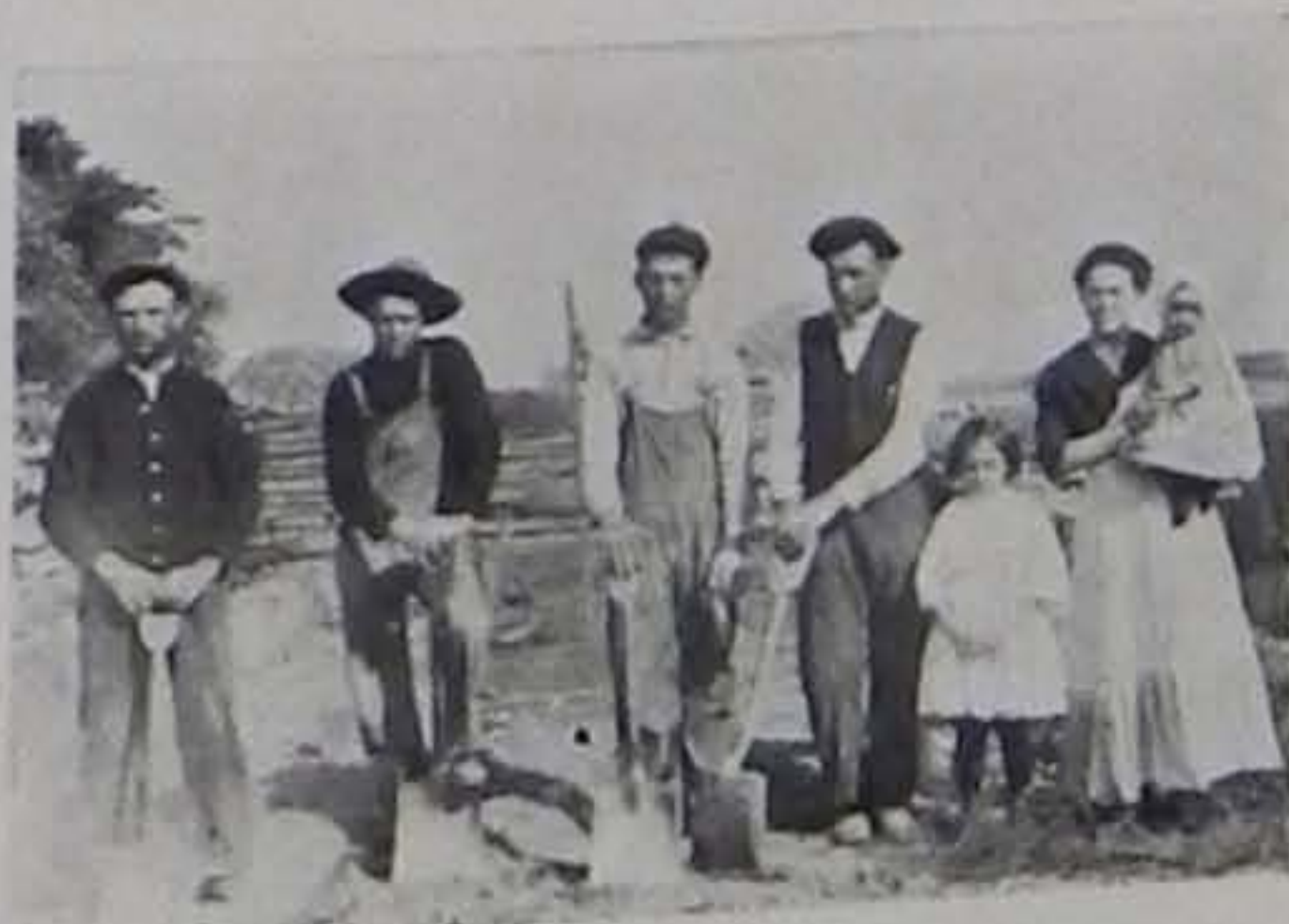
PHOTOGRAPH FROM J. R. DYER, Taken in 1912, while working on foundation for corn crib, LOVINGTON, ILL.
