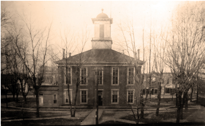
The Second Sullivan Court House
