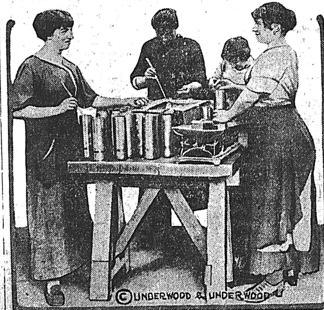
This photograph shows a scene now common in France, where the women have largely taken the place of men in the ammunition factories. They are seen filling shells with shrapnel.
